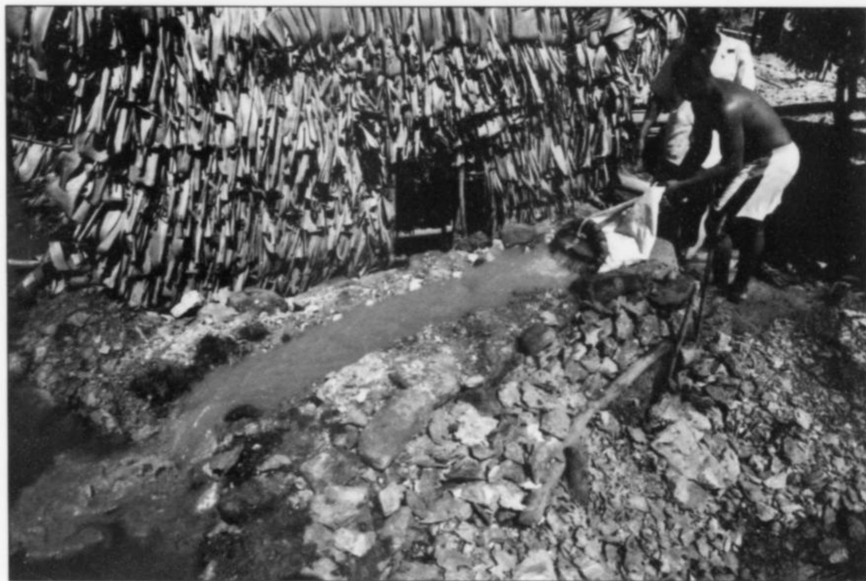
Figure 6. Water channel built to carry water away from a pit that is being drained. Robert Zawadzki photo.
