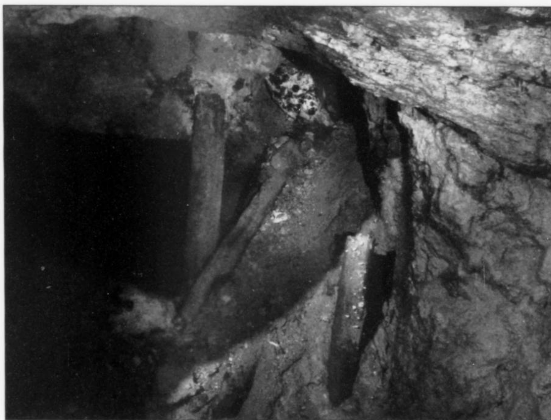
Figure 22. A cleft system cut by a tunnel in the Resplendor mine. Guido Steger photo.
