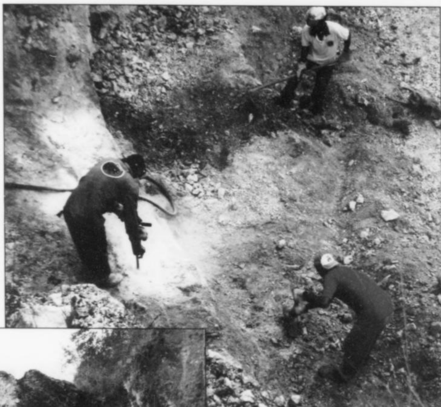
Figure 11. Miners at their work with jack drills on a steep slope of the Lavra Fazenda open cut. Guido Steger photo.
