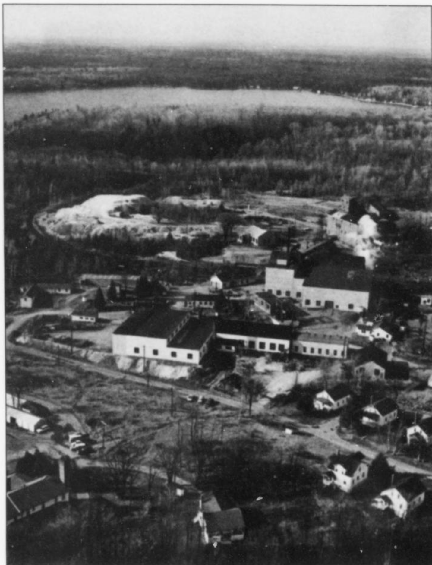
Figure 3. The Balmat mine processing facilities in 1963 (from the 100th Anniversary Annual Report of the St. Joseph Lead Company).
