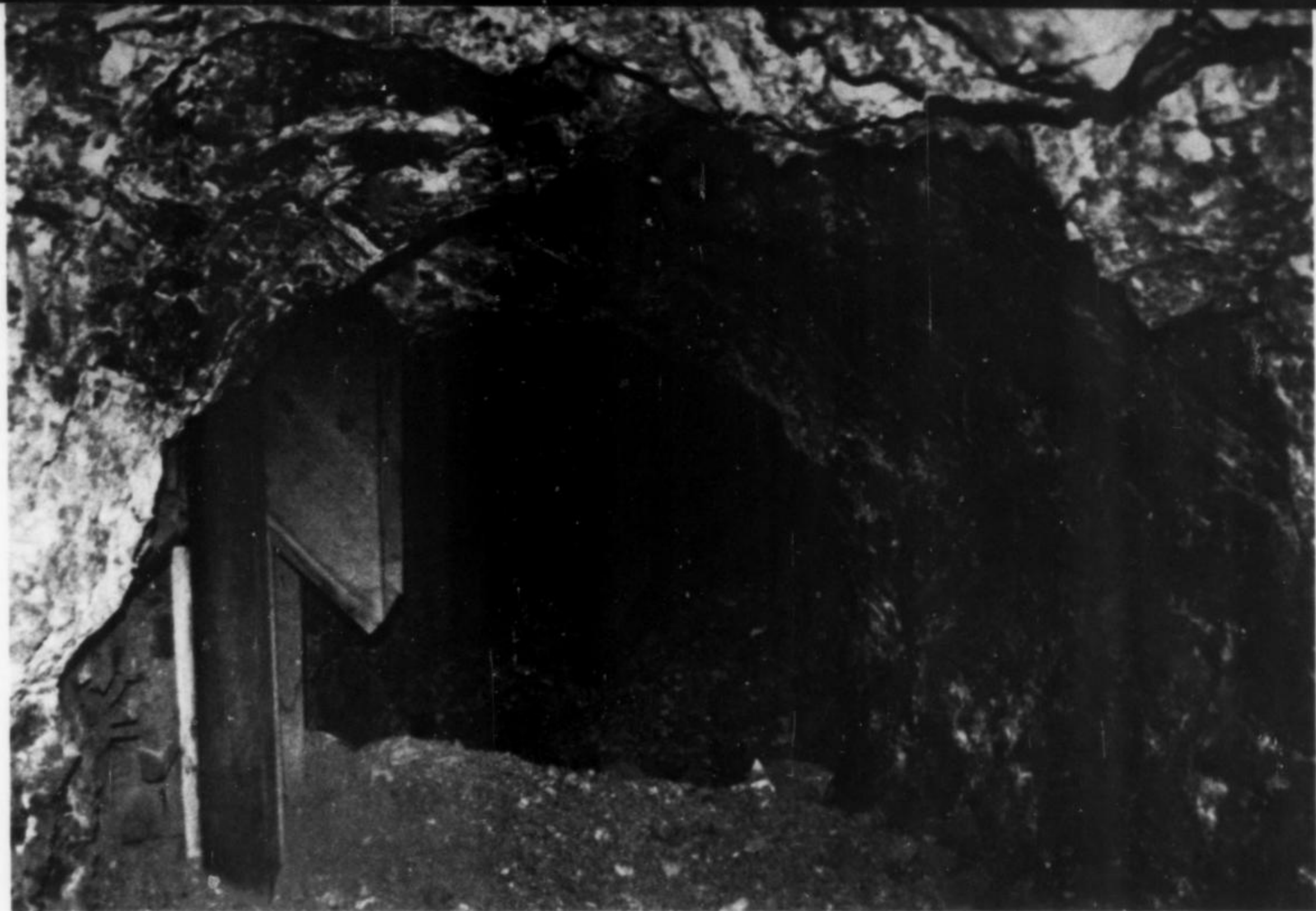
Fig. 7. The second and third ore chutes on the 100-foot level. The second chute (foreground) leads to the wulfenite stopes and the Jobes shaft.
