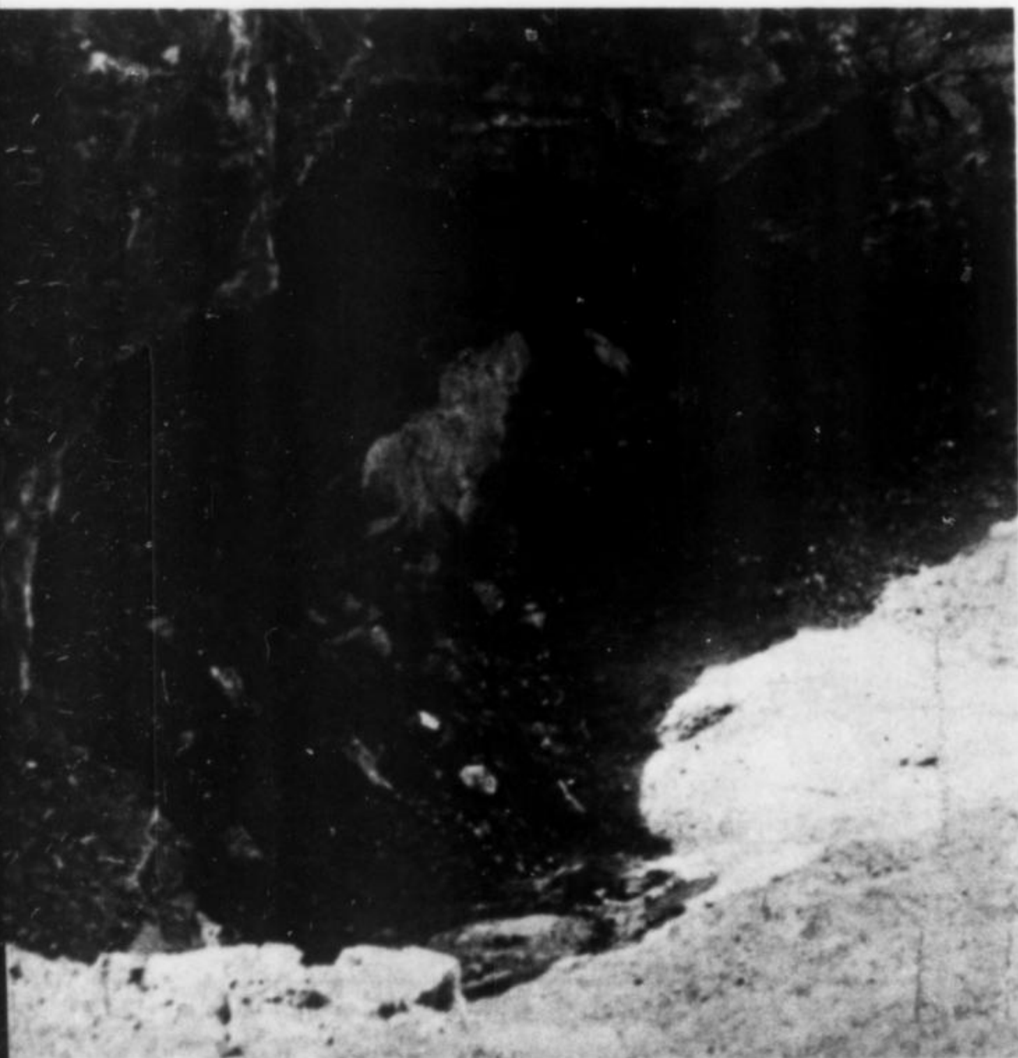
Fig. 6. Caved main stope of the Old Yuma mine, near Tucson, Arizona. The large block is about 20 feet across. This cave-in ended the productive history of one of the world's most famous vanadinite veins. Wulfenite can still be found elsewhere in the mine. No one is believed to have been in the mine at the time of the cave-in.
