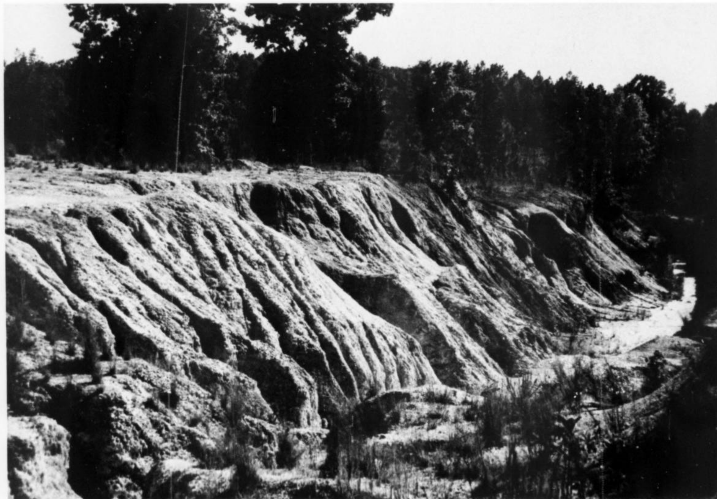
Fig. 2. The main trench on the Williams property. Weathering is ubiquitous; pegmatite weathers white, schist dark.
