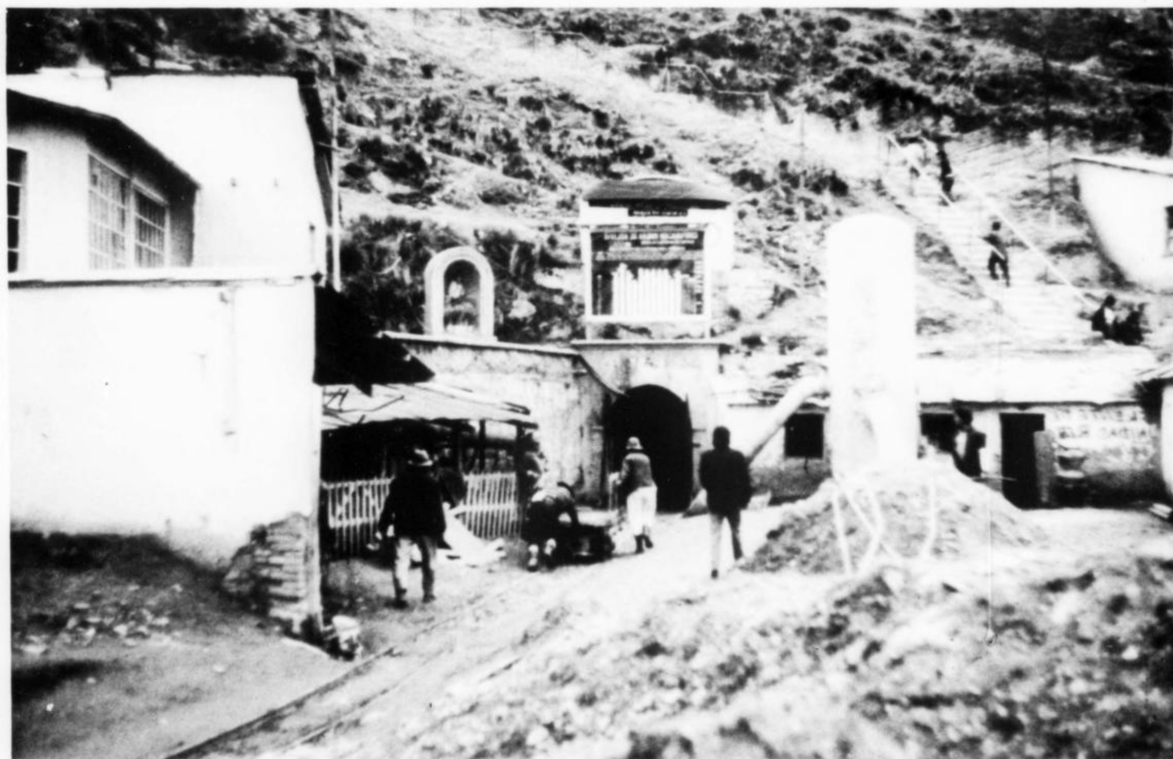
Figure 1. Main upper adit and mine office, Colquiri tin-zinc mine.
