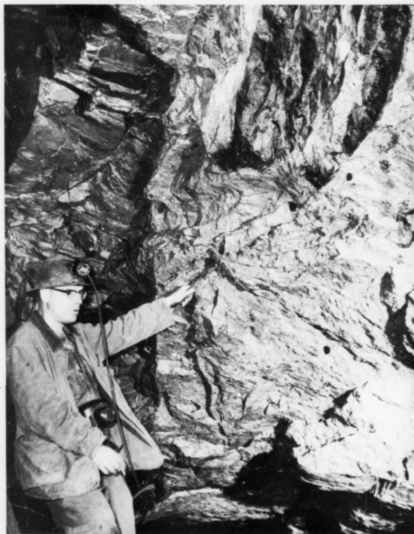
Fig. 3. (below) Hanging wall of massive millerite, 301-11-15 stope, No. 2 Mine.
