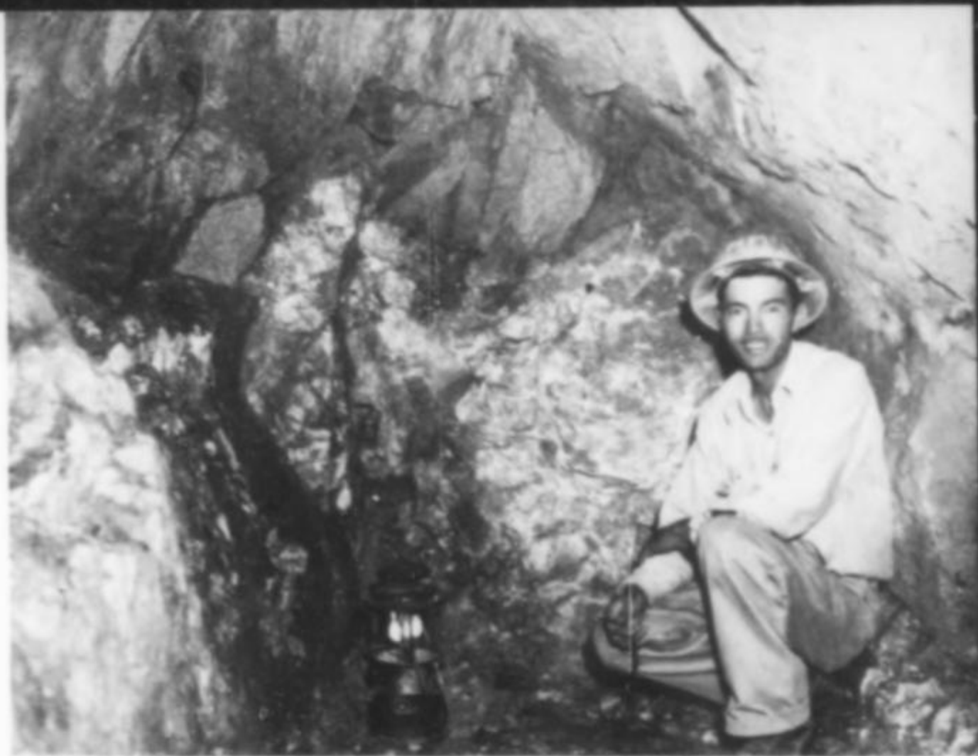
Figure 6. (above) Flaudio Griego at rich working face of a beryl tunnel, June 23, 1950. Small rolls in the pegmatite hanging wall are shown here in cross-section, with a thin, downward-projecting septum of country rock at left. At right the pegmatite body drops off abruptly on the flank of a large, asymmetric roll.
