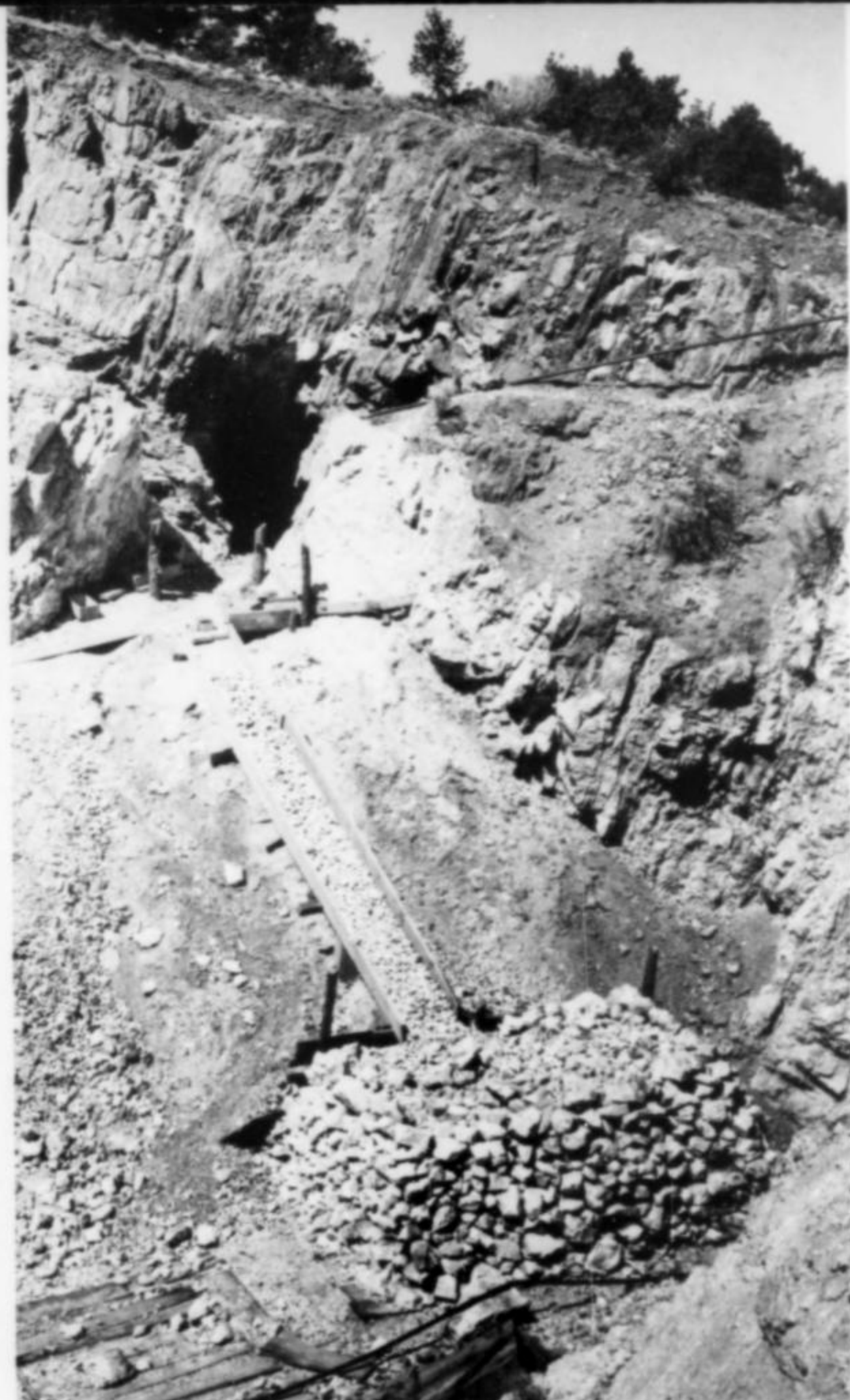
Figure 5. Portal of main beryl tunnel in hanging-wall pegmatite at west end of main quarry, June 1950. The stockpile in foreground represents four months of mining and hand sorting by three men.
