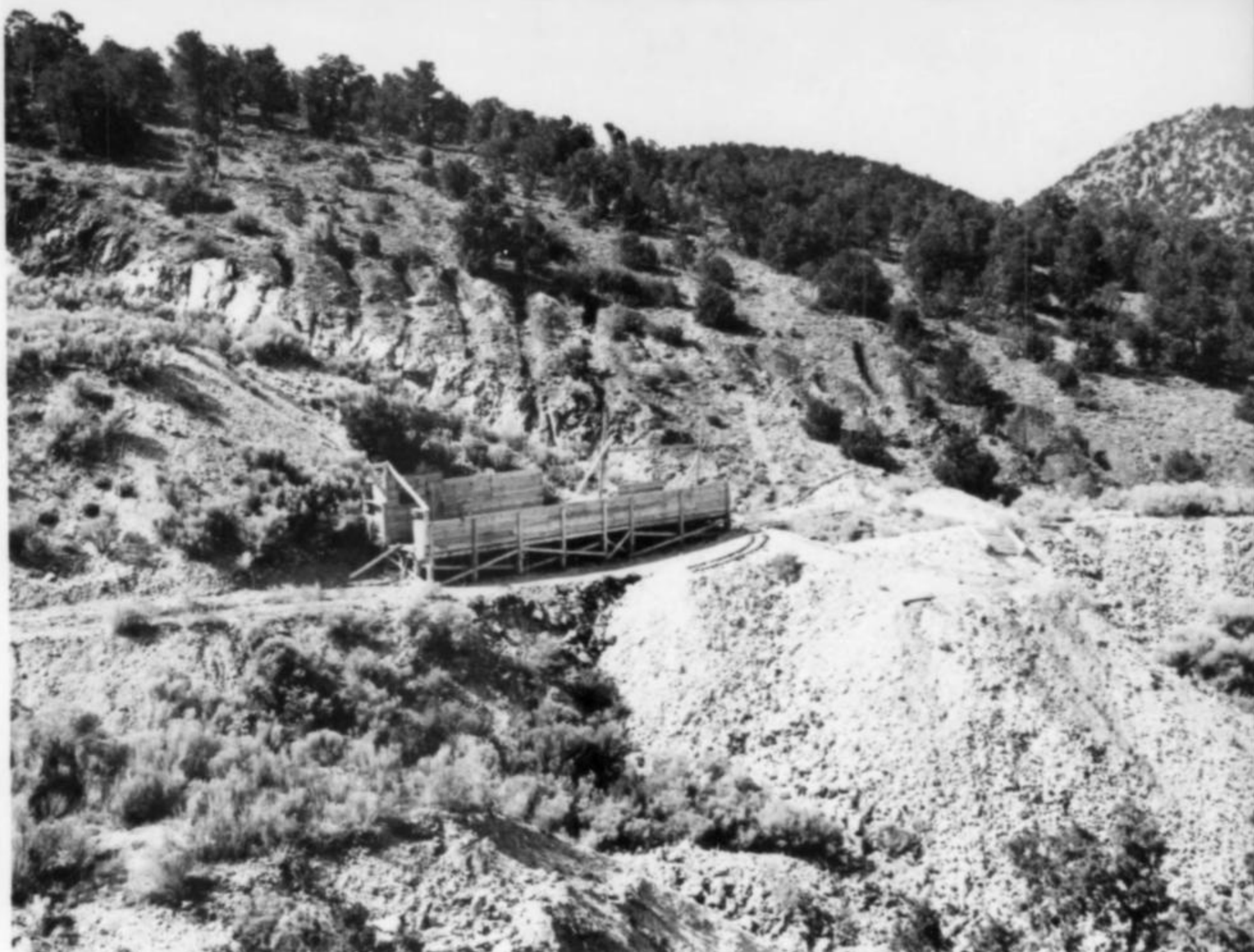
Figure 4. A 1943 southwestward view of west entry, some of the dumps from main quarry, and old platform for lepidolite ore. The parallel trenches on the hillslope were excavated by U.S. Bureau of Mines to expose the beryl-bearing upper part of the pegmatite body. The gently dipping contact between pegmatite (light) and overlying amphibolite (dark) appears high on the entry wall at upper left. The old dump in immediate foreground at left yielded the first microlite ore to be commercially recovered from the property (see Fig. 9).
