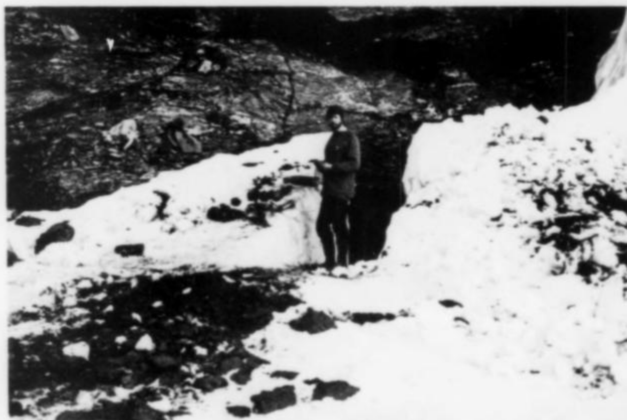
Figure 2. (below) Entrance to the tunnel. Note flat-lying foliation and abundant small quartz lenses in the phyllite. Scale: author (H.L.) is 190 cm (6'2") tall.
