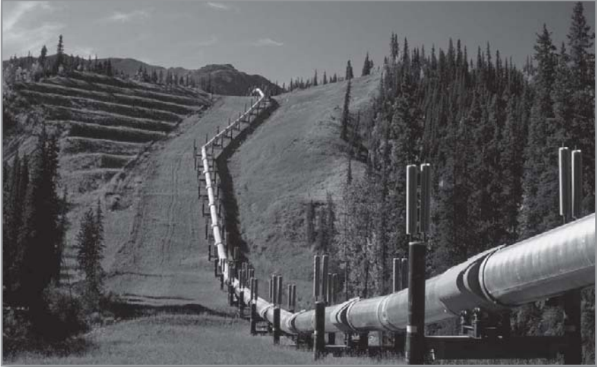
A length of the Trans-Alaska Pipeline near Squirrel Creek, Alaska. The pipeline was designed and built with the preservation of large areas of permafrost in mind. George F. Herben/National Geographic/Getty Images
