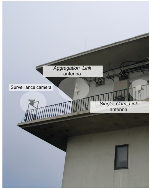
FIG. 32. Lousã Mountain surveillance tower: surveillance camera, subscriber station antenna ( Aggregation_Link SS), and base station antenna ( Single_Cam_Link ).
