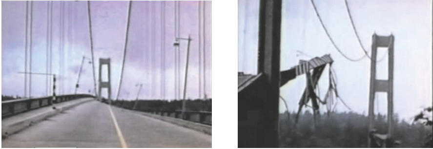
FIGURE 14 The Tacoma Narrows Bridge. Right picture is taken approximately 40 minutes after the left one.
