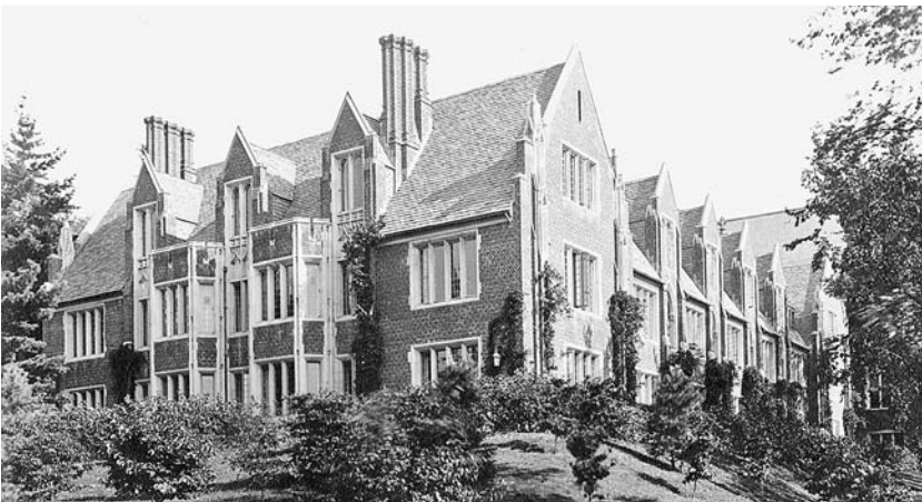
Henry Burchard Fine Hall at Princeton University, housing the Department of Mathematics (Princeton University Archives, Department of Rare Books and Special Collections)
