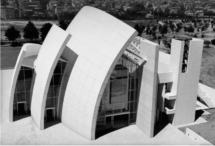
Fig. 29.10. The church of Dives in Misericordia , in Rome, built with a photocatalytic cement (Italcementi). Architect: Richard Meier
