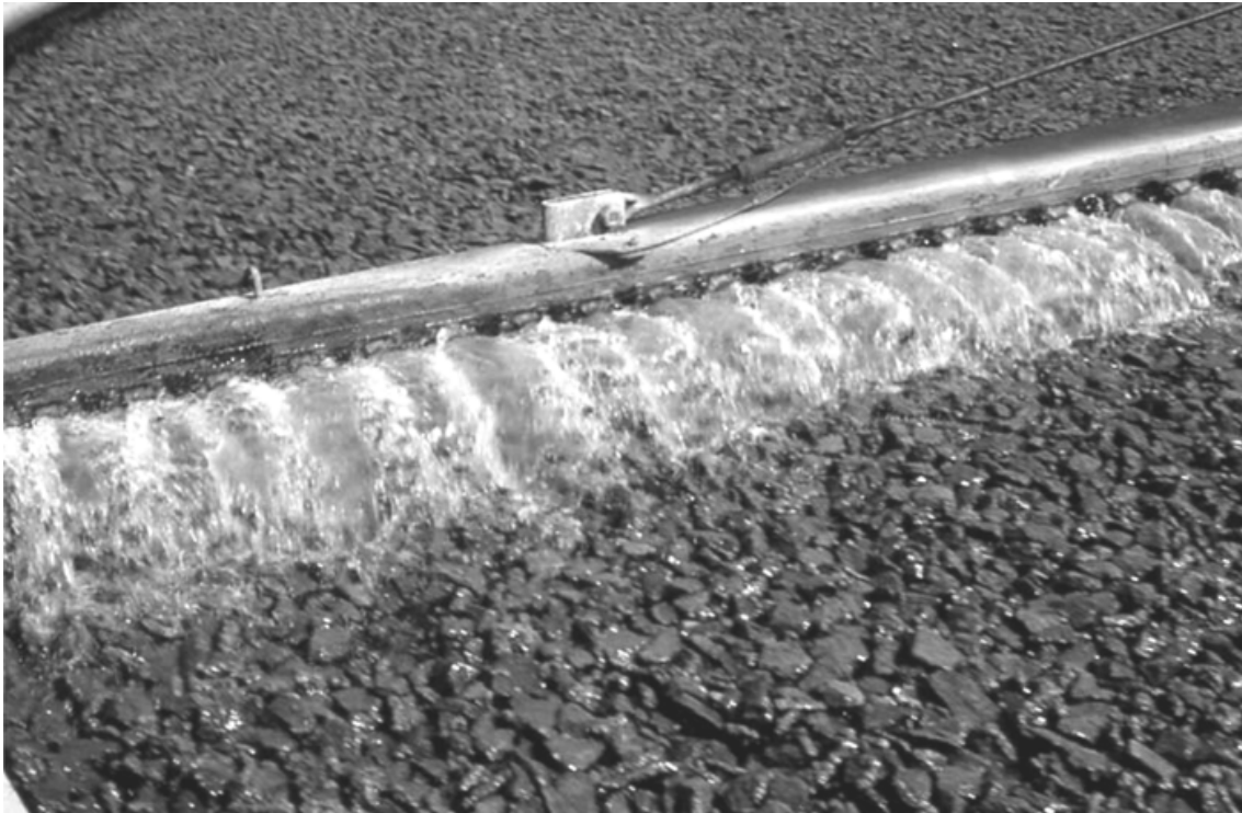
FIGURE 15.2 Trickling filter for use of wastewater treatment. The pebble stones are covered with microscopically visible microbial biofilms that mediate the degradation of organic and inorganic compounds. (Courtesy of Perry L. McCarty, Stanford University.)
