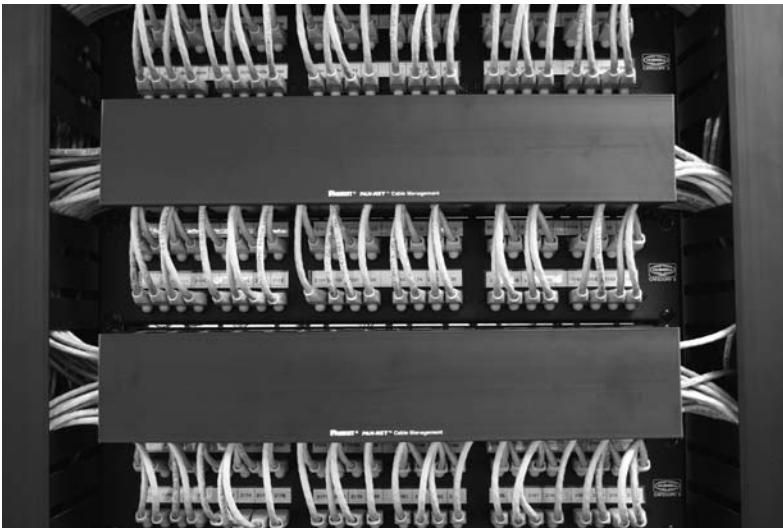
FIGURE C.1 Cable harnesses prevent excessive tangling by keeping associated wires bundled together.
