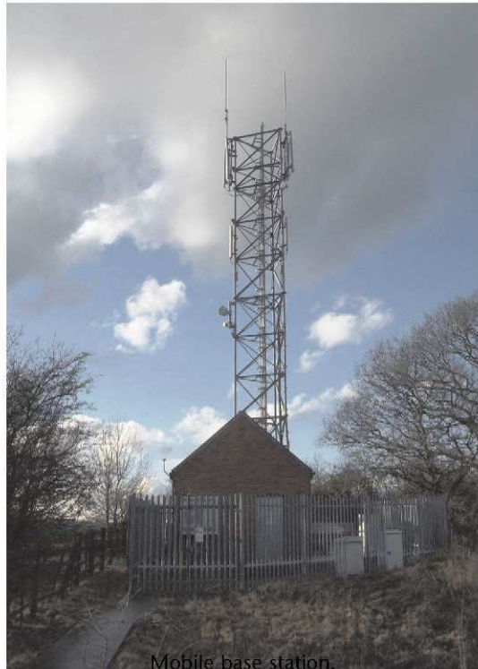
Mobile base station.
