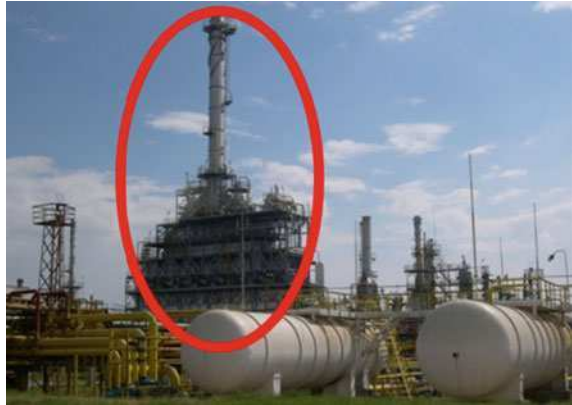
Fig. 4.9 Petroleum refinery plant
