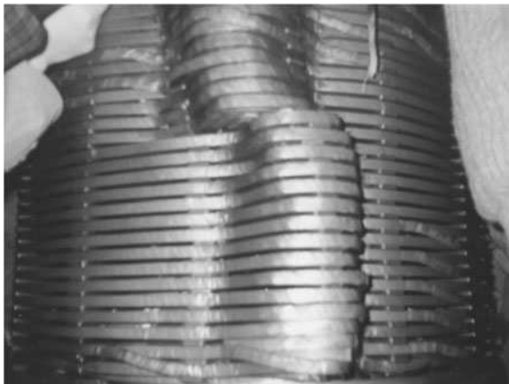
Fig. 9.1 A winding deformation fault found in a scrapped transmission transformer
