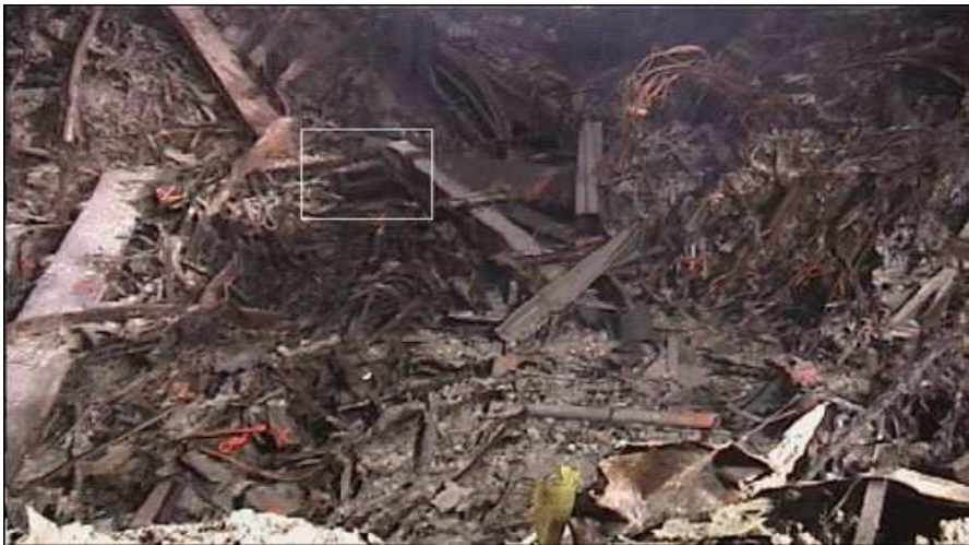
Fig. 3. The white square marks the entrance to a void searched, approximately 0.3 _ 0.5 m cross section (Casper, 2003)
