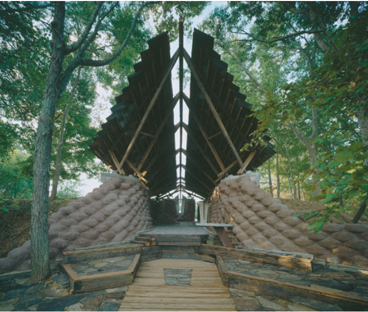
The Yancey Tire Chapel in Sawyerville, Alabama is a quintessential example of low-budget, experimental architecture. Student architects Steven Durden, Thomas Tretheway, and Ruard Veltman of Auburn University's Rural Studio constructed this striking chapel out of recycled tires, salvaged beams, tin, and rocks from a nearby river.
