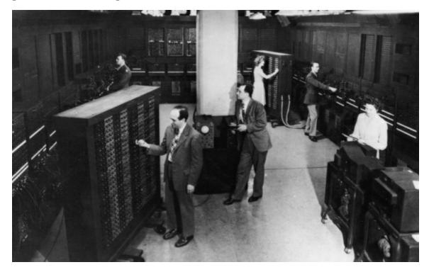
The ENIAC was able to solve many types of numerical problems – such as addition and subtraction. It was primarily used to calculate data for firing and launching weapons for the United States Army.
