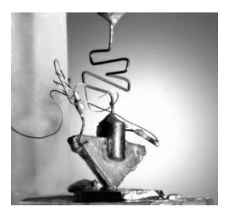
1947: Bell Labs invents the transistor (a device with no moving parts that can alter the flow of electricity in a machine).
