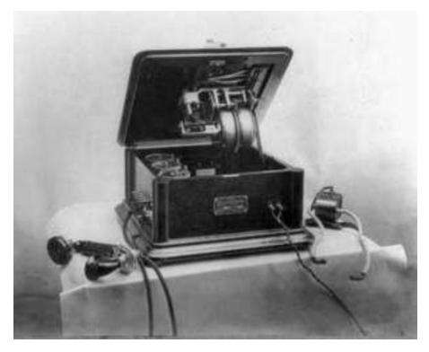
The telegraphone was able to record speech magnetically on a thin steel wire.
