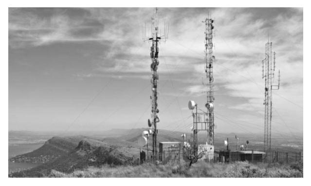
Each tower has a range around it in which it can send and receive data to various computer devices, as long as the device has the correct receiver and transmitter in it. Once you go beyond that range, the device and the tower can't detect each other anymore. In most places around the world now, before you pass out of the range of one tower, you pass into the range of a new tower.
