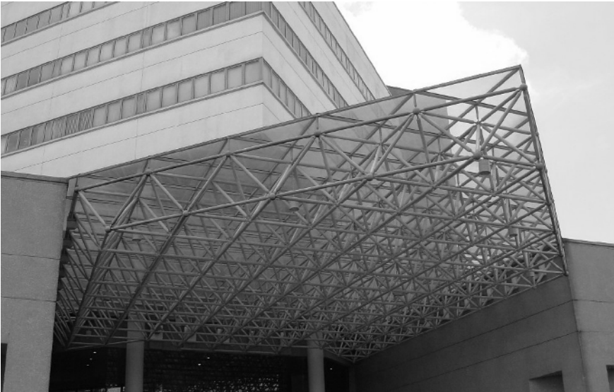
Figure 2.7. A typical structure made up of truss members. The entrance of the faculty of Engineering, National University of Singapore.
