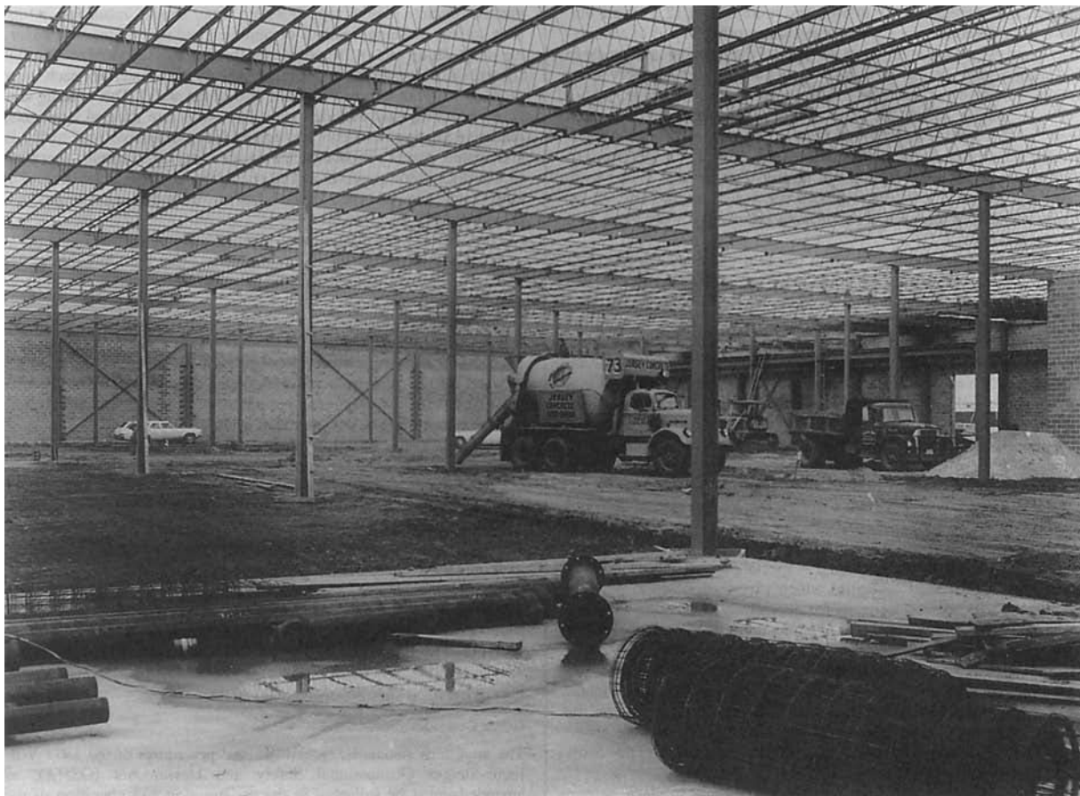
Fig. 12.1.10 A view of a plant during construction. Shown are its columns, roof trusses, and exterior masonry walls. The reinforced-concrete floor slab is being poured over compacted soil. (Source: VMA, Inc.)
