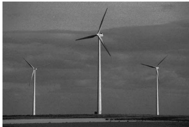
Figure 9.1.9c Wind turbines rated at 1.5 MW with 72-m-diam rotors at TVIG's Kimball wind farm installation in Nebraska. (Photo courtesy of Tennessee Valley Infrastructure Group Inc.)
