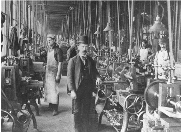
FIGURE 1.14. A photo showing early factory conditions during the industrial revolution.
