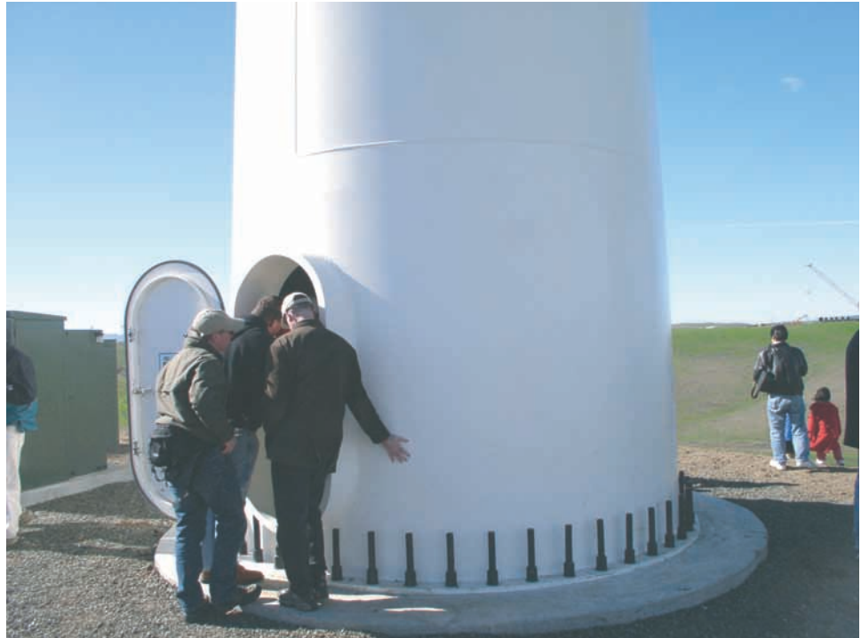
FIGURE 1.24. Entering the maintenance hatch in one of the Solano wind turbine towers. Courtesy of D. K. Lieu
