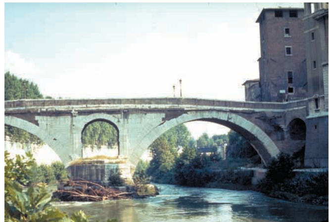
FIGURE 1.04. Pont-du-Gard Roman aqueduct (left) built in 19 BC to carry water across the Gardon Valley to Nîmes. Spans of the first- and second-level arches are 53–80 feet. The Ponte Fabricio bridge in Rome (right) built in 64 BC spans the bank of the River Tiber and Tiber Island.
