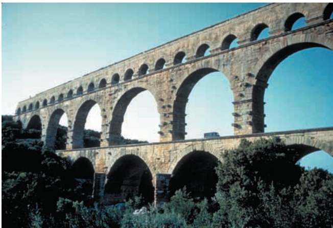
FIGURE 1.04. Pont-du-Gard Roman aqueduct (left) built in 19 BC to carry water across the Gardon Valley to Nîmes. Spans of the first- and second-level arches are 53–80 feet. The Ponte Fabricio bridge in Rome (right) built in 64 BC spans the bank of the River Tiber and Tiber Island.
