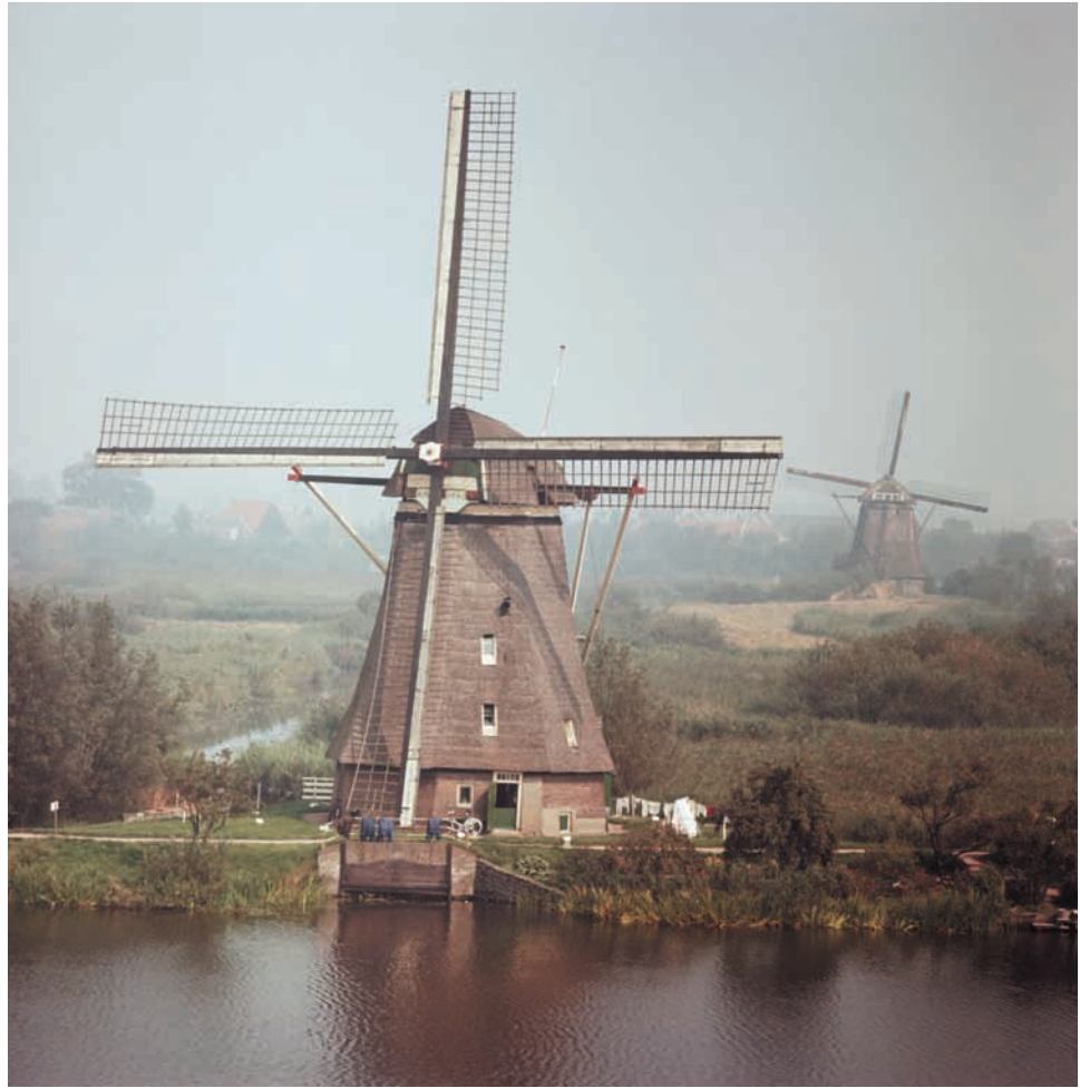
FIGURE 1.09. The network of windmills in Holland, used to drain water from flooded land, is an example of an early large-scale civil engineering project. Source: © PaulAlmasy/CORBIS
