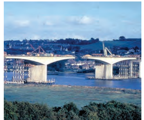
Photo 5.2 Nonprismatic cantilever beams of bridge during construction.
