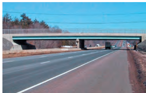
Photo 9.3 The continuous beams supporting this highway overpass have three supports and are thus statically indeterminate.
