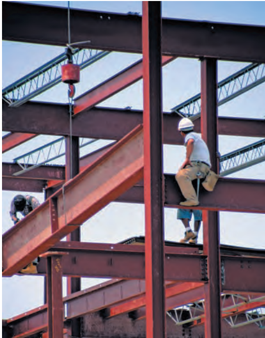
Photo 4.3 Wide-flange steel beams form the frame of many buildings.
