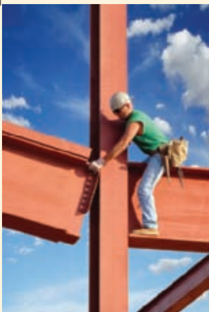
Slender steel column with lateral support near mid-height (Lester Lefkowitz/Getty Images)
