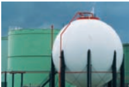
Thin-walled spherical pressure vessel used for storage of propane in this oil refinery (Wayne Eastep/Getty Images)
