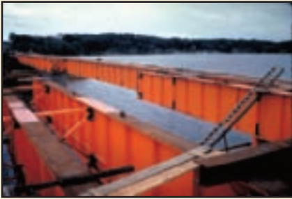
Beam with overhang loaded by gravity uniform load (Courtesy of the National Information Service for Earthquake Engineering EERC, University of California, Berkeley)
