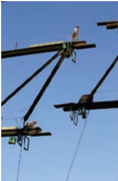
Forces can develop in statically indeterminate trusses due to temperature and prestrain (Barros & Barros/Getty Images)
