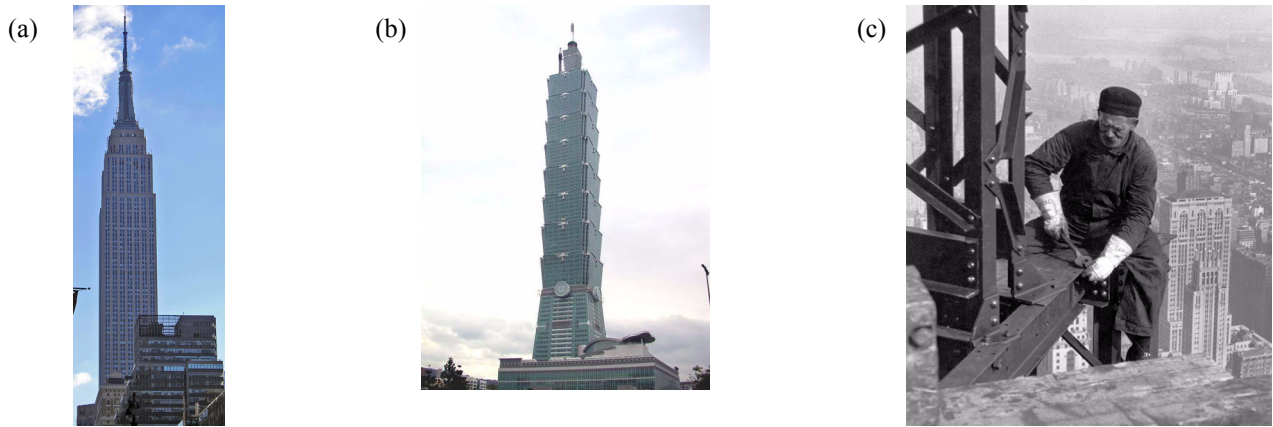
Figure 7.25 (a) Empire State in New York. (b) Taipei 101 in Taipei, Taiwan. (c) Joint construction.
