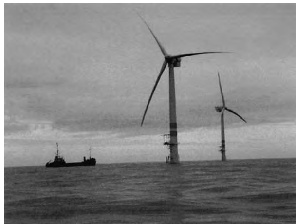
Figure 9.1.9d Located about 10 km off the coast of Arklow, Ireland, the Arklow Bank offshore wind park consists of seven GE Wind 3.6-MW wind turbines. Construction was completed in 2003. (Photo: Robert Thresher.)
