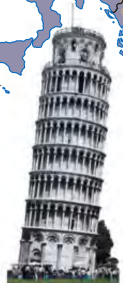
Leaning Tower of Pisa, a famous tilting building in Pisa, Italy.
