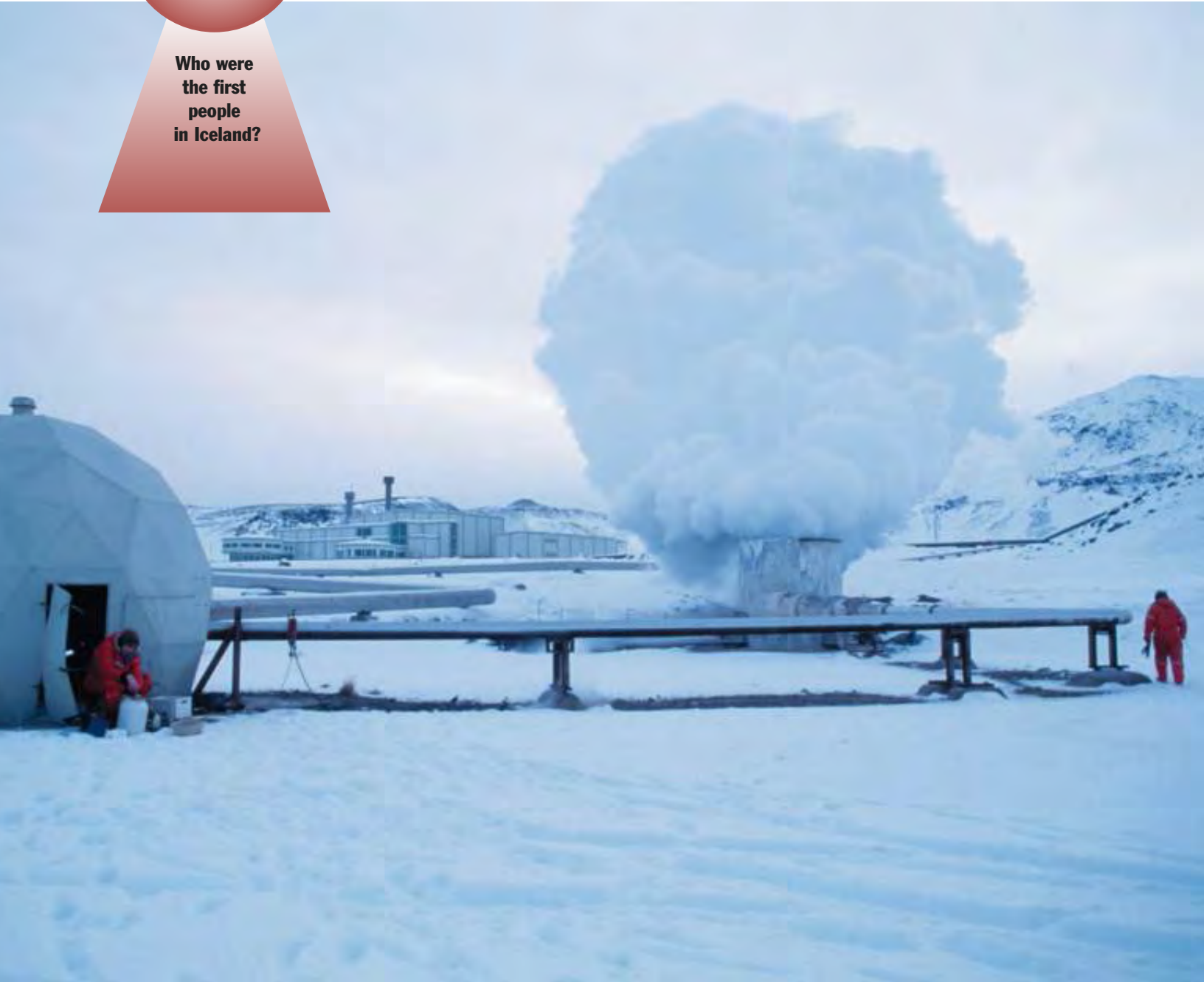
This power plant produces heat for the city of Reykjavik using steam from hot springs. © Roger Ressmeyer/Corbis
