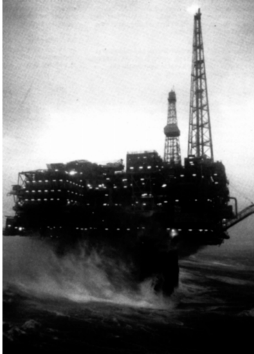
Plate 2. Oil platform in rough seas (the North Sea basin).
