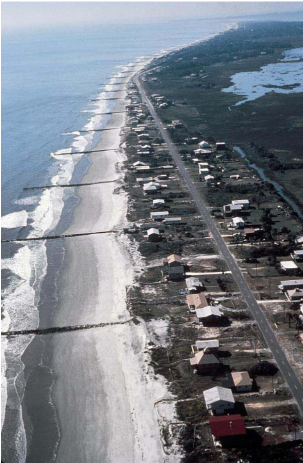
Figure 6 A groin field along Pawleys Island, South Carolina. Trapping of sand on the updrift side of a groin, and erosion of the beach on the downdrift side usually results in a sawtooth pattern to the beach. Note that in this example the beach is the same width on both sides of each groin, indicating little or no longshore transport of sand.
