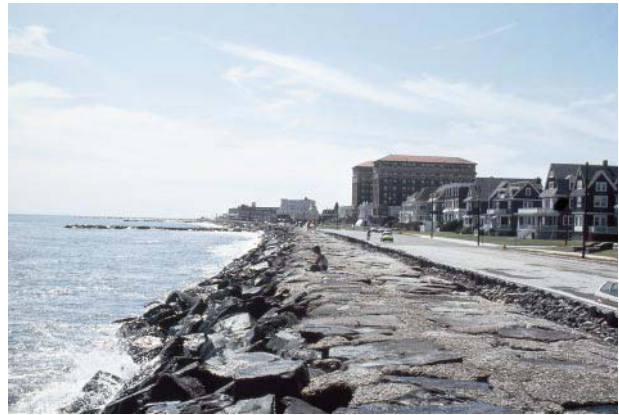
Figure 4 Cape May, New Jersey has been a popular seaside resort since 1800. Several generations of larger and larger seawalls have been built as coastal erosion caught up with the older structures. Today in many places there is no beach left in front of the seawall.
