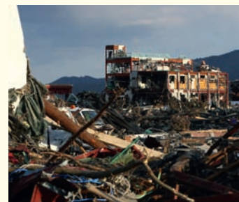
Damage from the 9.0 earthquake and resulting tsunami, northern Japan, March 2011.
