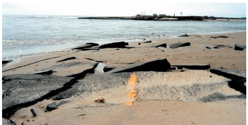
(c) The breach severed the only road along the island's length and isolated many homes. The arrow in (b) and the yellow line in (c) mark the centerline of the road.
