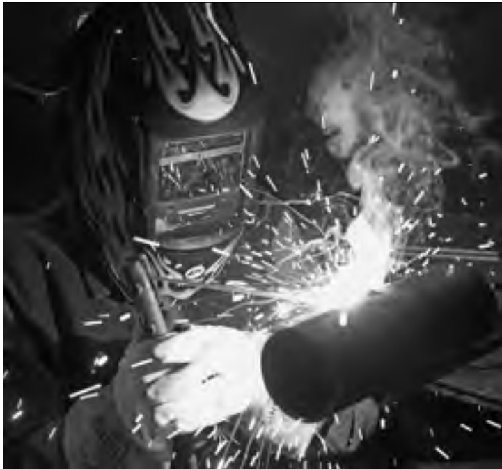
Figure 14-1: Steel pipe being stick welded.
