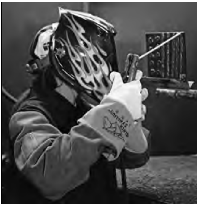
Figure 6-5: Practicing vertical-up welding.
