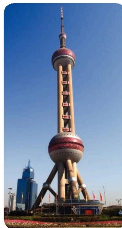
▲ The Oriental Pearl Tower in Shanghai is over half a kilometre high. In high winds, its top can move by a quarter of a metre. But, being elastic, its steel and concrete structure always returns to its original shape.
