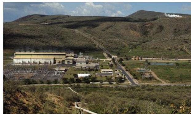
↑ Pipes are buried deep in the rock below this geothermal power station.
