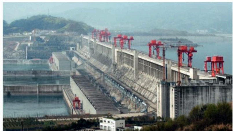
This hydroelectric dam has a power output of millions of watts. Some dams are large enough to provide enough electricity for a large city
