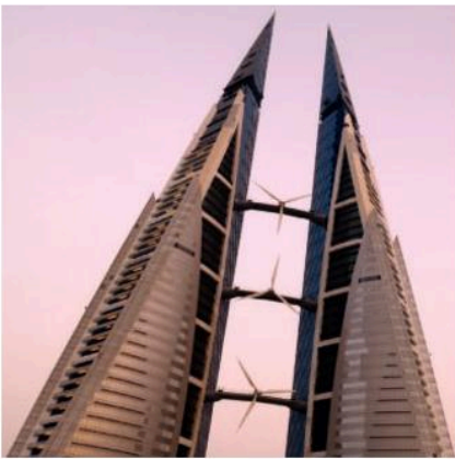
The world trade centre building in Bahrain has several wind turbines built into its structure. The turbines produce up to 15% of the electricity requirements of the building
