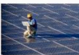
An engineer tests the output of a large array of photovoltaic cells.
