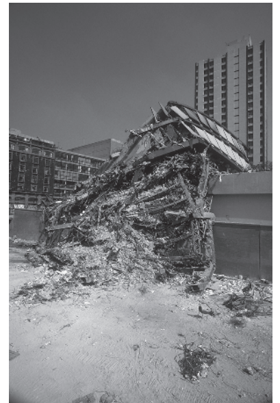
FIGURE 13.26 Oscillations of the ground during an earthquake can drive resonant oscillations in buildings whose natural frequencies include those of the earthquake oscillations. This helps explain why some buildings collapse while neighboring buildings sustain only modest damage. Photo shows the aftermath of the 1985 magnitude-8.1 earthquake in Mexico City.
