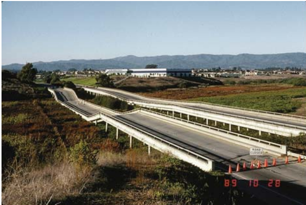
FIGURE 10.6 One result of the 1989 earthquake near San Francisco, CA. The earthquake vibrations overlapped with the suspended highway resonant frequencies causing large amplitude vibrations leading to its collapse.
