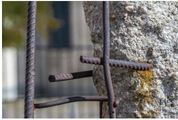
Figure 10.5 Remnant of the Berlin Wall. The fourth and final stage of construction (1975–1980) employed about 45 000 slabs of reinforced concrete. Each slab was 3.6 m tall and 1.2 m wide. ©Steve Tulley/Alamy
