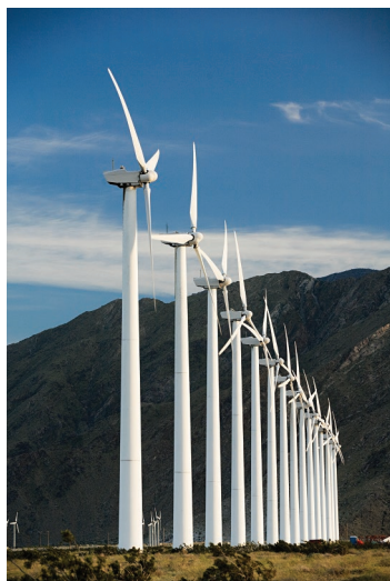
Figure 6.1 At a California wind farm, these wind turbines convert the energy of motion of the air into electric energy.
