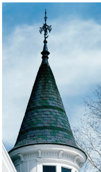
Figure 16.47 An elaborate lightning rod protects a Victorian house in Mt. Horeb, Wisconsin. ©Paul McMahon/Heartland Images
