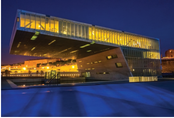
Figure 8.20 Villa Méditerranée in Marseille, France, designed by architect Stefano Boeri. A cantilevered exhibition space extends 40 m out over a 2000 m 2 pool and offers panoramic views of the sea. ©Provence/Alamy
