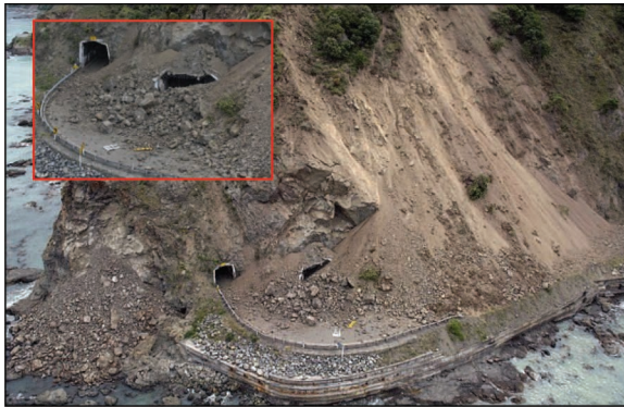
Figure 2.2 A major landslide near Kaikoura (South Island). (Source: en.wikipedia.org.)
