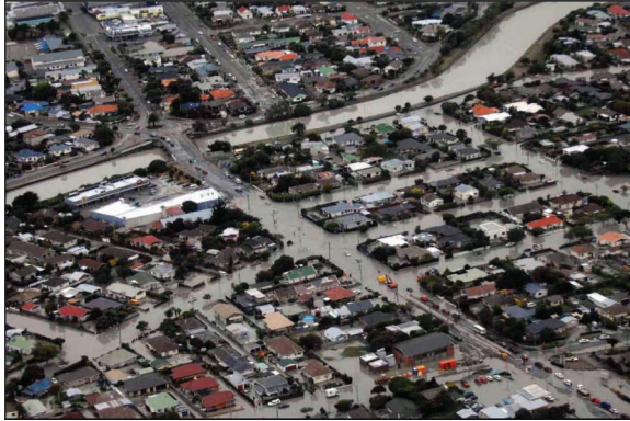
Figure 2.3 Aerial view of liquefaction-affected areas in Christchurch city. (Source: en.wikipedia.org.)
