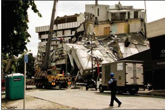
Figure 2.1 Destruction of the Pyne Gould building in Christchurch city. (Source: en.wikipedia.org.)
