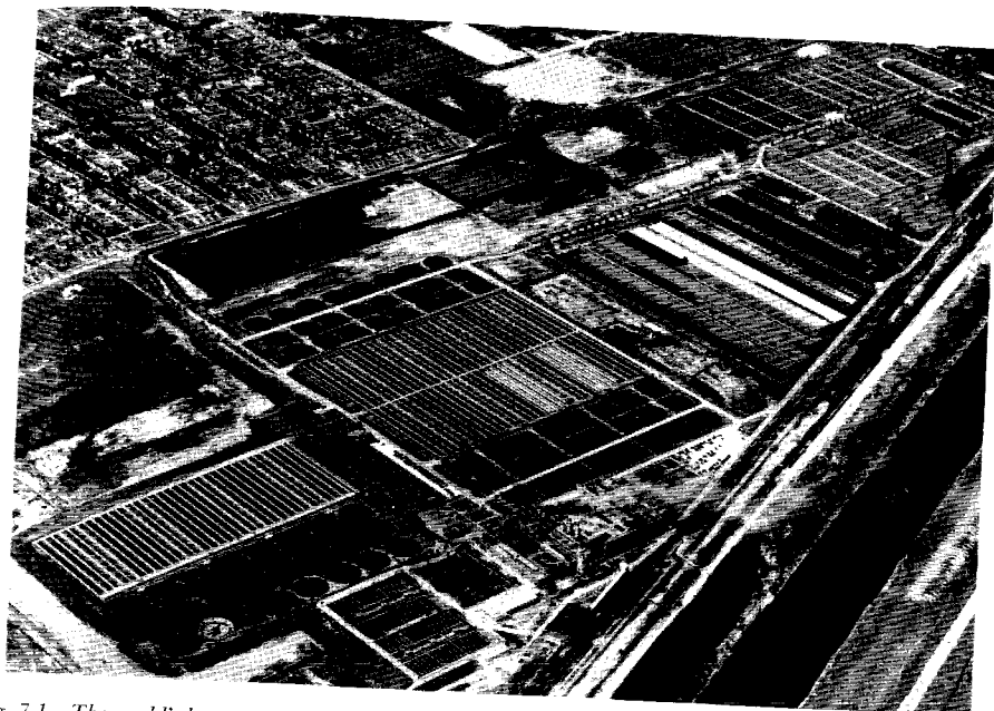
Fig. 7.1. The world's largest sewage treatment system at Chicago has been termed by the American Society of Civil Engineers "the seventh wonder of America." More than 1,100,000,000 gallons of waste are treated daily in the system. In this view can be seen the preliminary settling tanks, the aeration tanks, and the final settling tanks. Each of the final settling tanks is 126 feet in diameter. (Chicago Aerial Industries, Inc.)
