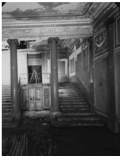
Fig. 1 Foyer of the theatre, right side, after the fire
