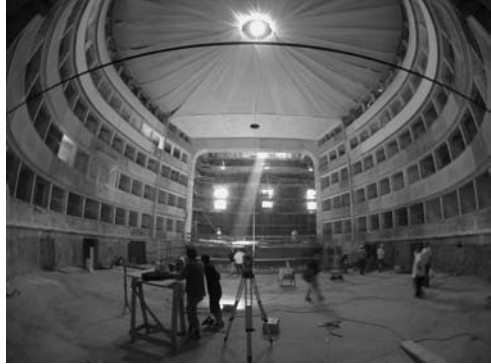
Fig. 6 Theatre auditorium, June 2003: restored wooden structure of the boxes
