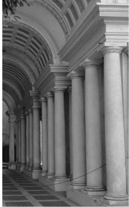
Fig. 9 Oblique deformation of the architectural orders in the perspective gallery of Palazzo Spada, Rome
