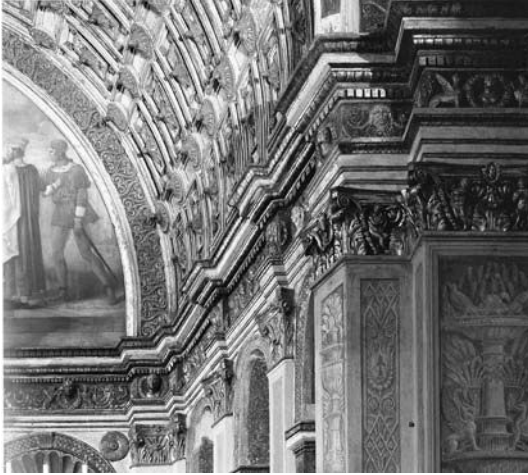
Fig. 10 Oblique deformation of the architectural orders in the fake choir of Santa Maria presso San Satiro, Milan
