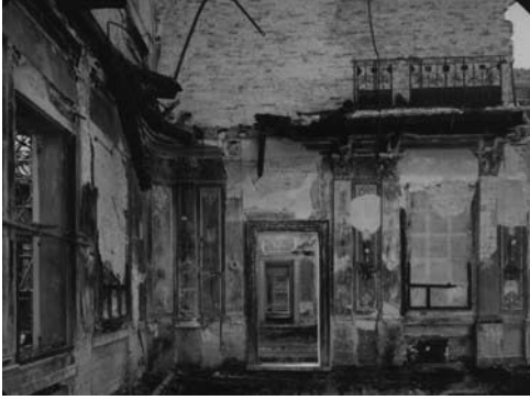
Fig. 3 Sala Grande after the fire
