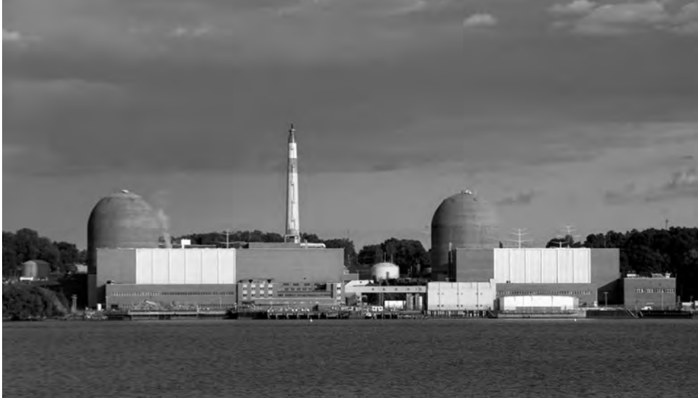
The Indian Point Energy Center on the Hudson River in New York state uses nuclear fission to heat water and produce steam. Except for the fuel source, nuclear power plants operate just like any other type of power plant.
