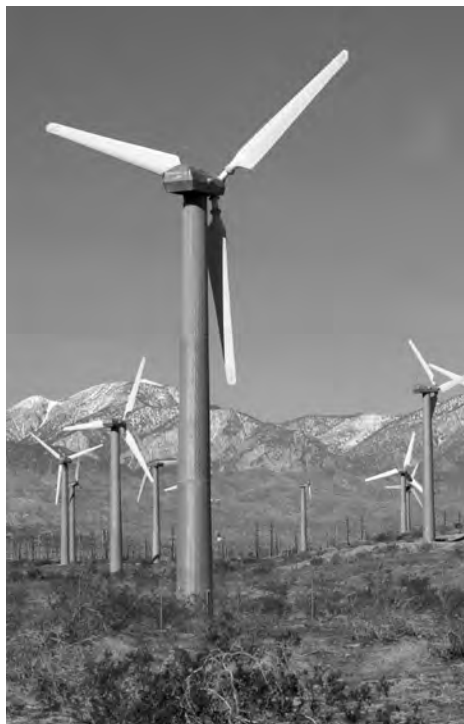
Windmill blades may move slowly, but they can produce a lot of torque. Gears increase the rotational speed but reduce the torque, driving an electric generator. Almost all the energy from the wind is delivered to the generator.
