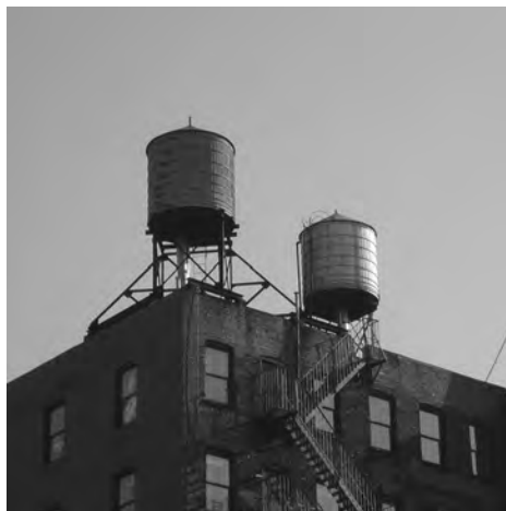
Water towers such as these in New York City are often placed on top of tall buildings. This way, the force of gravity supplies the water pressure needed to deliver water throughout the building.
