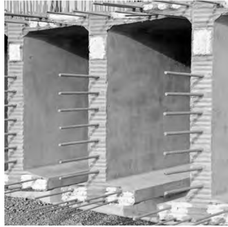
Reinforcing concrete blocks with rebar (steel bars) helps support the concrete and keep it from cracking. Composite materials such as these blocks are an example of how combining materials that have compressive strength with those that have tensile strength is an effective strategy in construction.
