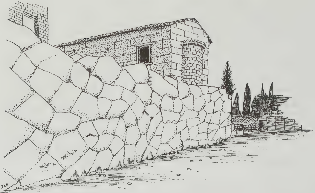
Polygonal stonework at an ancient fortified site in northeastern Greece. There is a superficial resemblance to Incan stonework. (R7)
