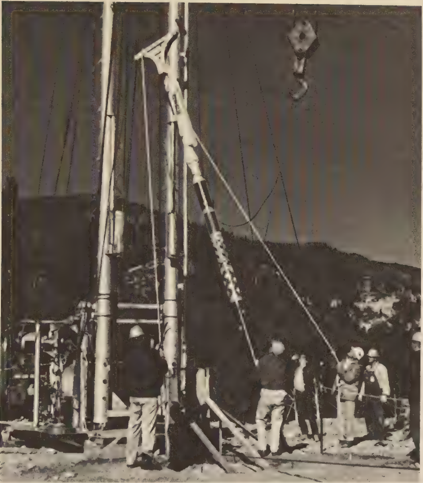
The Project Rulison 30-kiloton nuclear charge is shown being lowered into the shot hole near Rifle, Colorado, in 1969. (U.S. Atomic Energy Commission)
