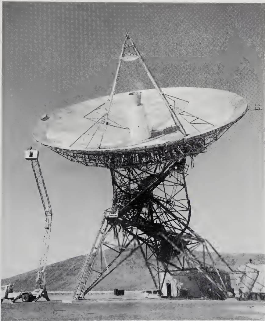
Fig. 6-15. The 26-meter (85-ft) paraboloid antenna at the JPL Goldstone station. (Courtesy of the Jet Propulsion Laboratory)
