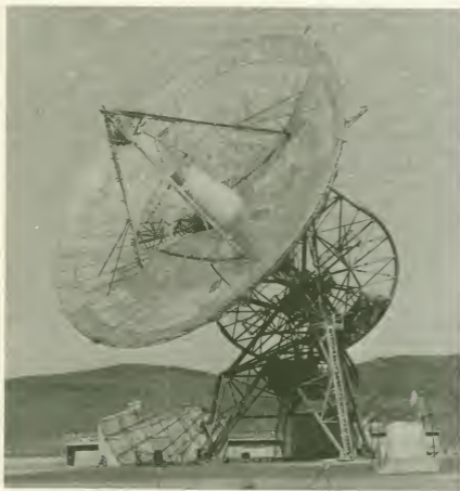
FIGURE 8-1.—The first 85-ft paraboloidal antenna installed at Goldstone (Pioneer site).
