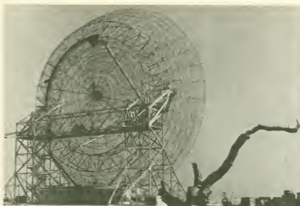
FIGURE 5-21.—The 150-ft dish at Stanford University, Palo Alto, Calif. This antenna is used in the radio propagation experiment.
