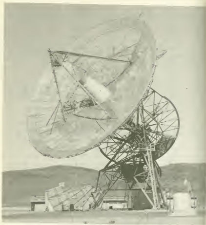
FIGURE 2-26.—The first 85-ft paraboloidal antenna installed at Goldstone (Pioneer site).
