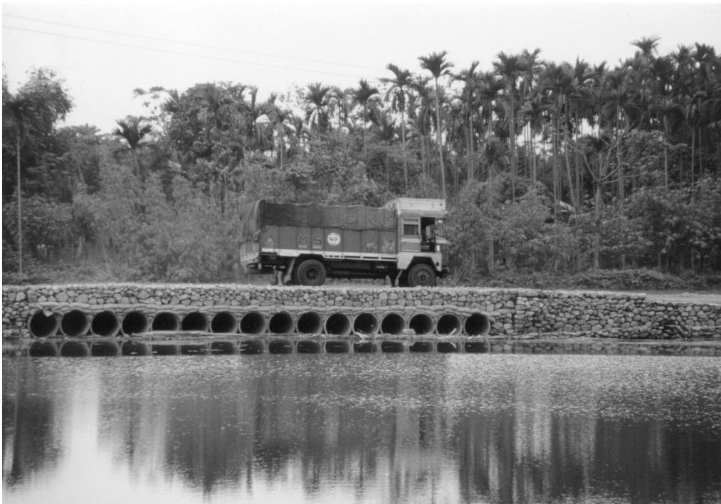
Multiple culvert in India. (Photo: Bent Thagesen)
