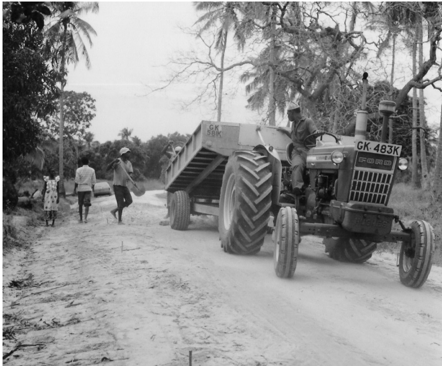
Figure 18.4 Gravelling rural access roads in Kenya. Photograph courtesy of TRL Ltd.
